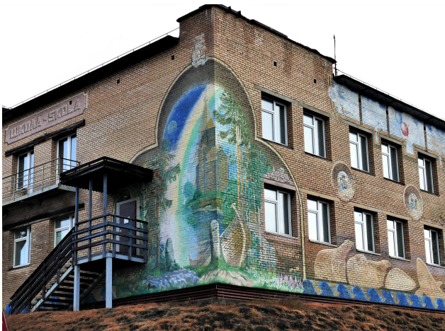
Figure 10. School building of Barentsburg (photo: B. Schennerlein).
